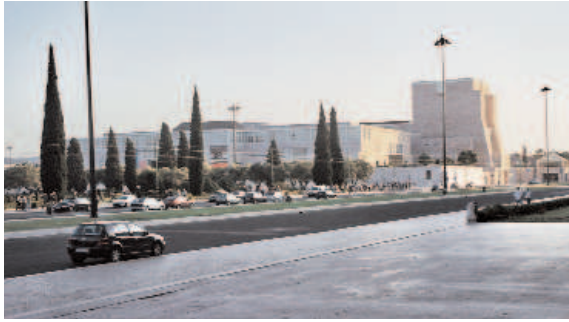
Belem conference centre (front)
